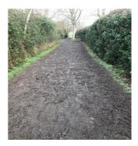
The access at the southern end onto common lane also has considerable trip hazards caused by the uneven surface and tree roots in the gap adjacent to the stone stile. The small trees/bushes need cutting back and the roots removed (pic 3)
